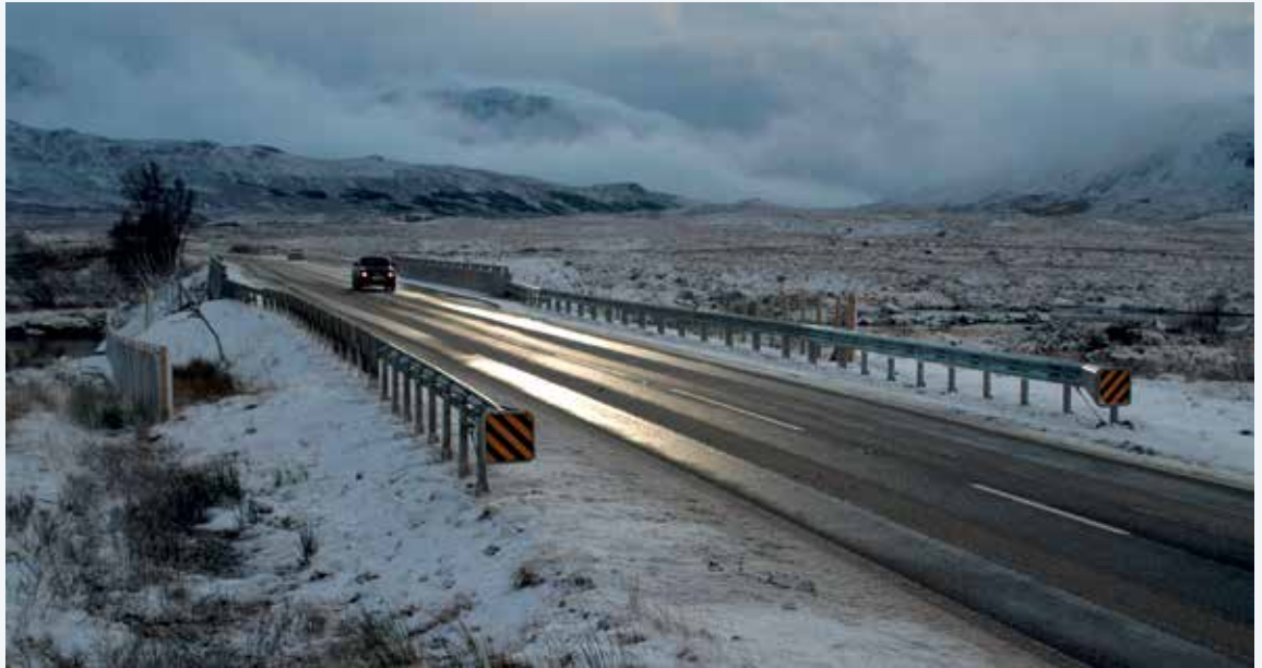
Hill and Smith's road safety products in use in Scotland; the company provides galvanising services and offers a wide spread of infrastructure-related products to an increasing number of international markets.
